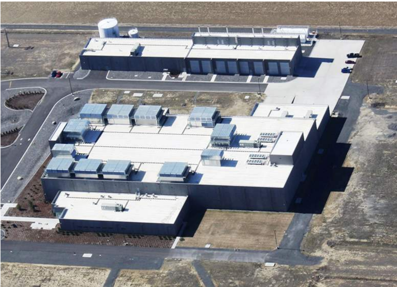
Dell Data Center in Quincy
